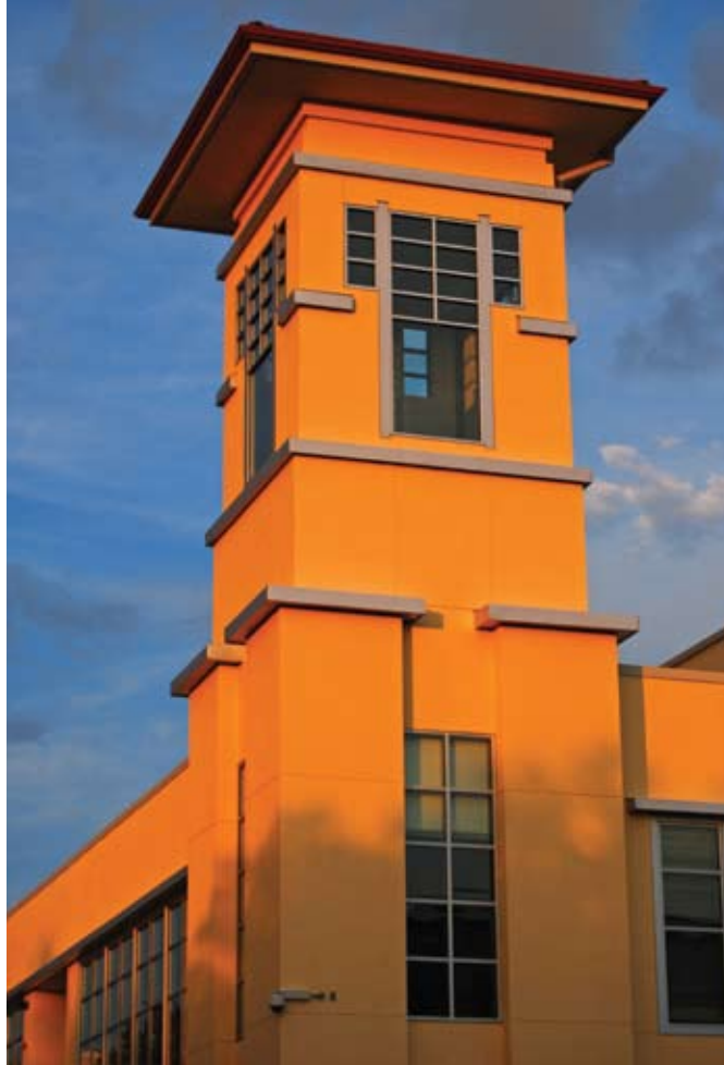
The University of Texas—San Antonio (new building) University Center San Antonio, Texas
