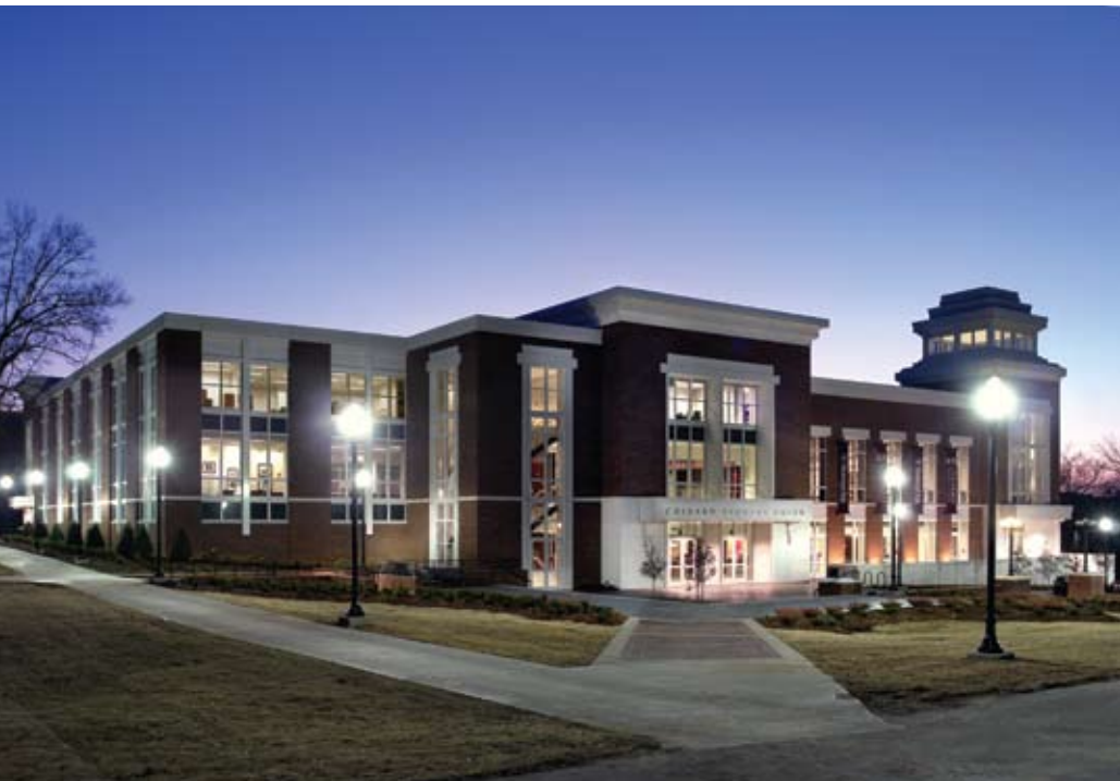
Mississippi State University (renovation/addition) Colvard Student Union Mississippi State, Miss.
